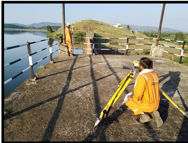
Level transfer from Fuse Gate to OBS KAKDIAMBA
