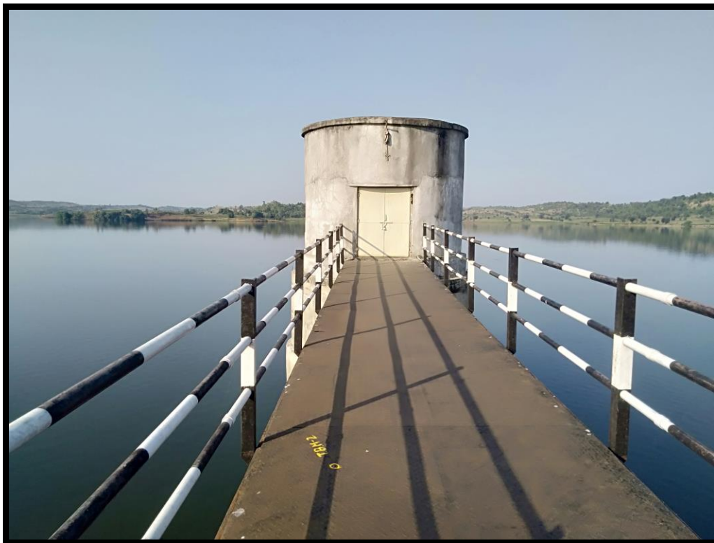
Control Cabin and TBM 2
