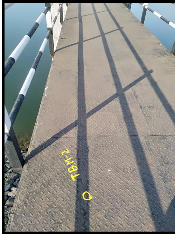
TBM 2 on near Control cabin
